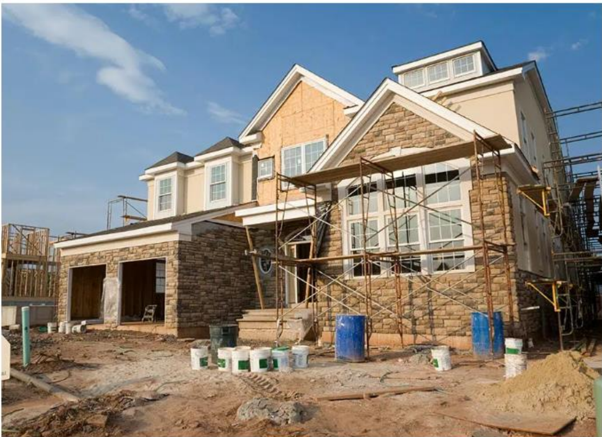
A LARGE HOUSING DEVELOPMENT BEING COMPLETED
